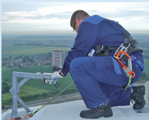
Installation Feuer W, rot
